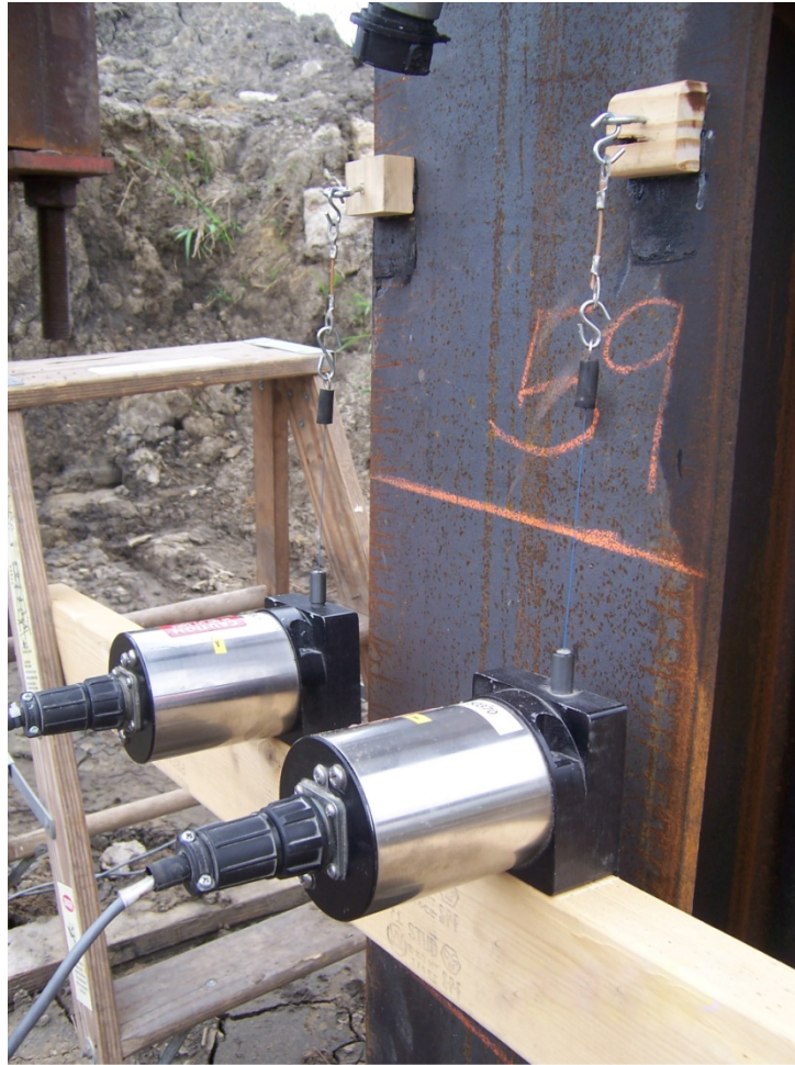
Figure 4.12: Displacement Transducers and Eye Hooks Mounted to the ISU4 Test Pile
