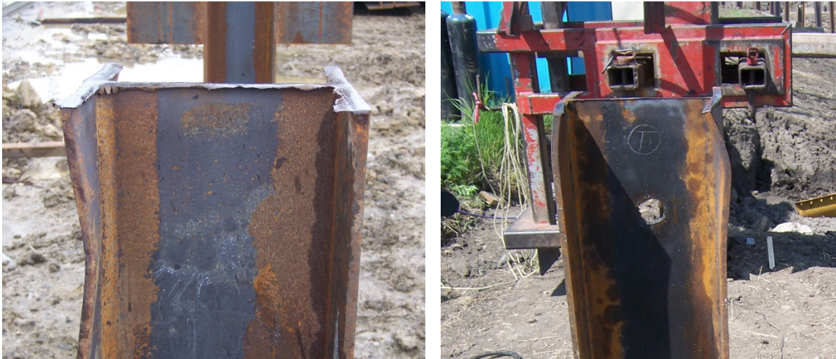
Figure 4.4: Local Buckling Damage of Test Pile Flanges for ISU5 (Left) and ISU8 (Right) due to Pile Driving
