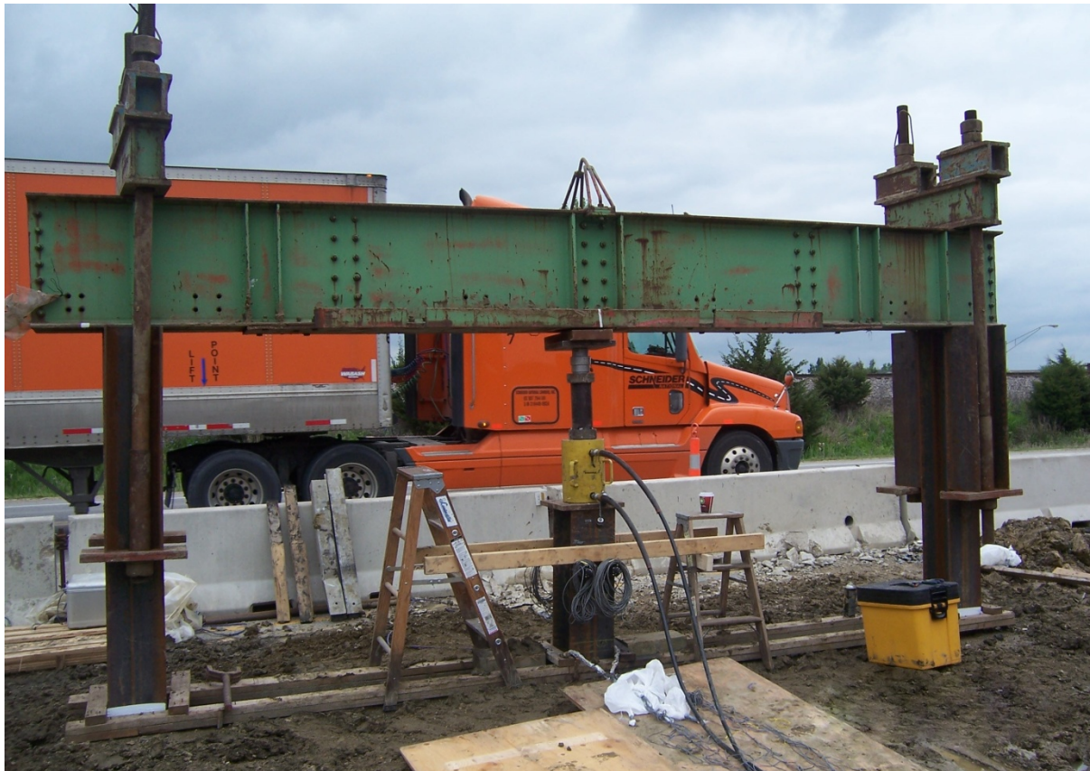
Figure 4.10: Completed Vertical Load Test Setup used for ISU5
